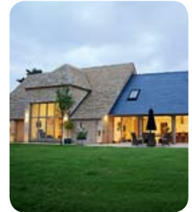
400-year-old barn goes eco Barnsley Hill Farm by Stonebee Developments ( stonebee.co.uk )
